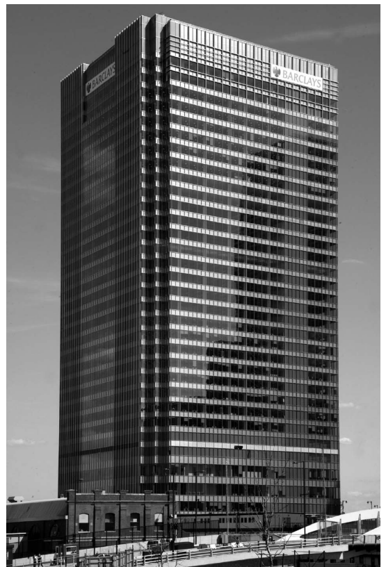
Barclays Group Headquarters, 1 Churchill Place
